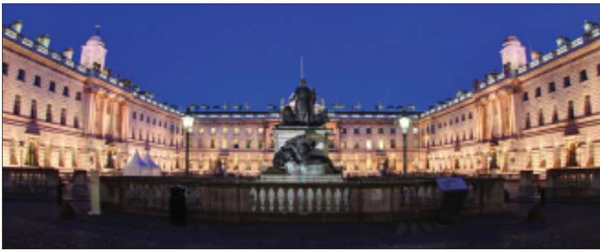
Above: Somerset House, one of the lighting installation achievements of AC Special Projects.
